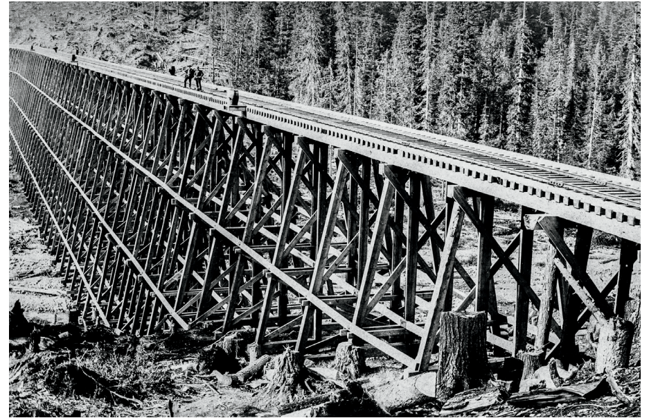
The second crossing of Loop Brook was the longest on The Loops. This view is west (railway-east) toward Ross Peak, whose slopes were the vantage for the image below. Note the water barrels on the trestle (explained on the following page), and that some of the timbers have not been uniformly milled.
