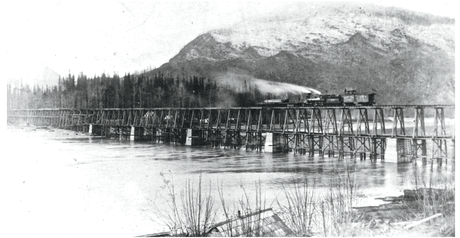
In this view from 1885, locomotive 46, a cordwood-fired 4-4-0, Standard American-type, built in 1882, hauls a flatcar of timbers over the first bridge at the “Second Crossing” of the Columbia River near Revelstoke. The present-day bridge is the fourth at that location and dates to 1968.
