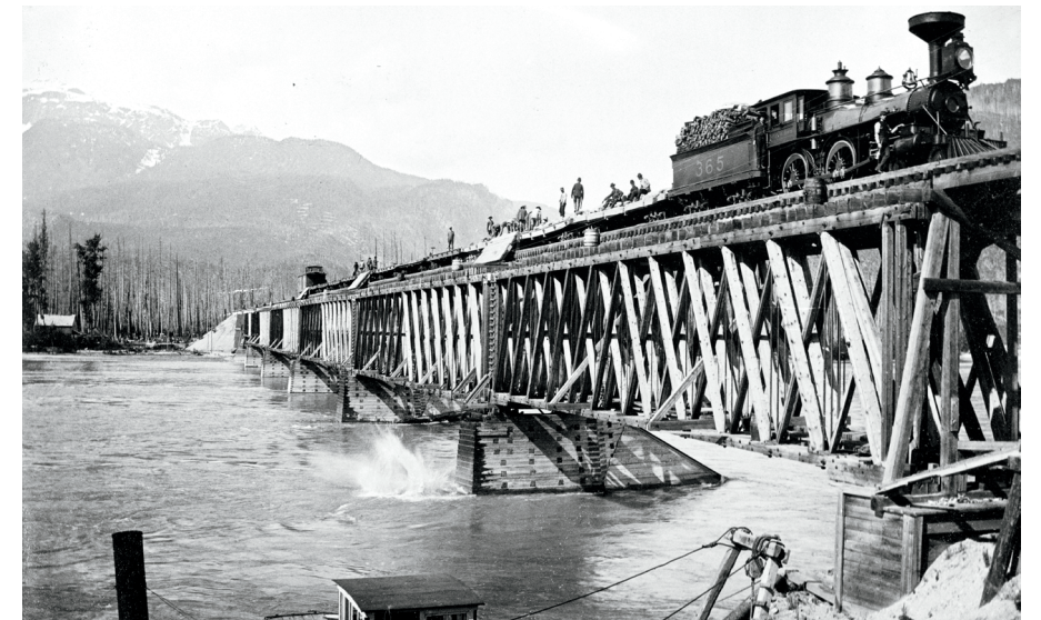
The second construction of the “Second Crossing” bridge is nearing completion as cordwood-fired locomotive 365 heads a work train, dumping fill to shore the footings. 365 was also a Standard American-type, built in 1886. Later renumbered 120 when converted to coal, and then renumbered 7073, it saw service for more than 40 years despite being avalanched in Rogers Pass in 1886. (See p. 72.) By 1899, the second span of this bridge had been modified to allow stern-wheelers to pass beneath.
