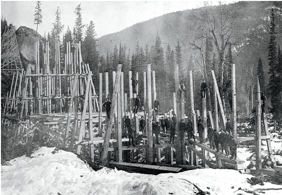
Construction of the Mountain Creek bridge began in the dead of winter, early in 1885.
