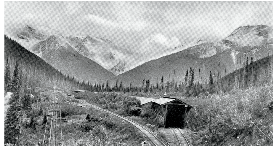
This is the same scene approximately 18 years later. A jungle-like growth of alder, willow, and other shrubs masks the construction scars. The buildings of the first Rogers Pass station are long gone.
