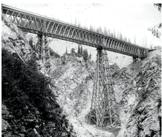
Stoney Creek bridge 1890
